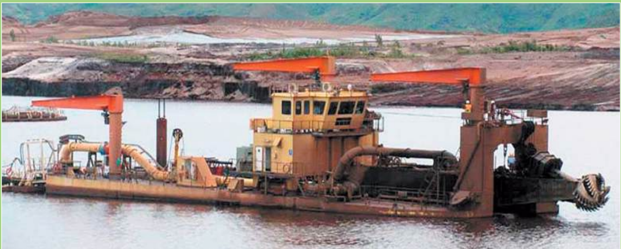
The timing of the mine-path taken by the floating dredge was altered to reduce impacts on local ecosystem services: forest products used by local communities.
