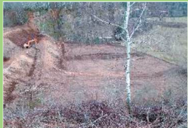
Soil stripping and vegetation clearance being undertaken in winter, outside the bird nesting season
